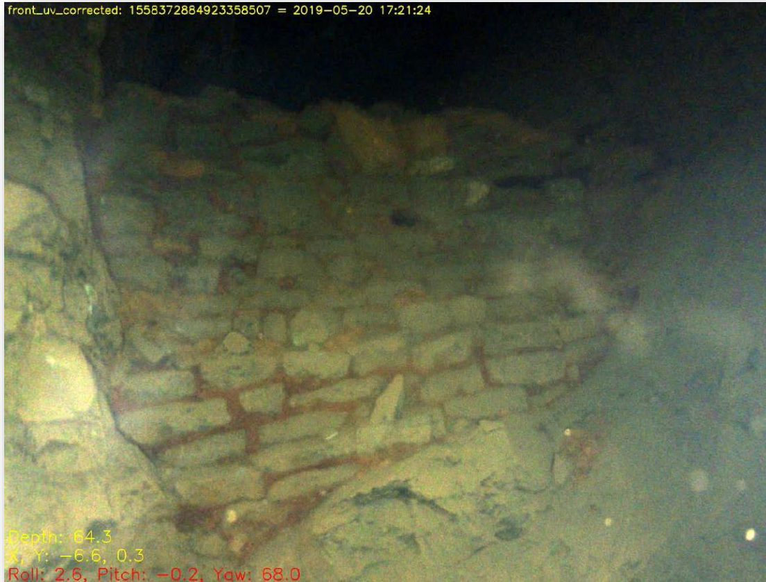
Built dam in the pumping shaft (-64 m)
